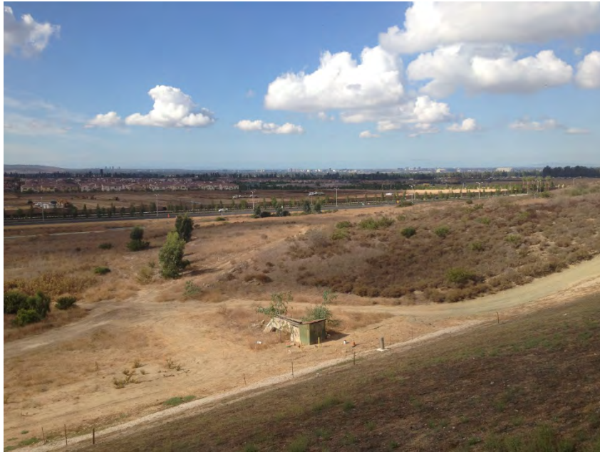
Exhibit A – Photograph is facing northwest and represents the project site (dam face is in the foreground)
