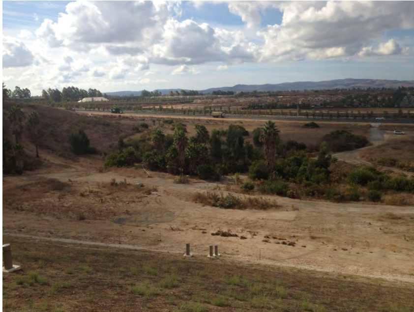
Exhibit C – Photograph is facing southwest and represents the project site (dam face is in the foreground)
