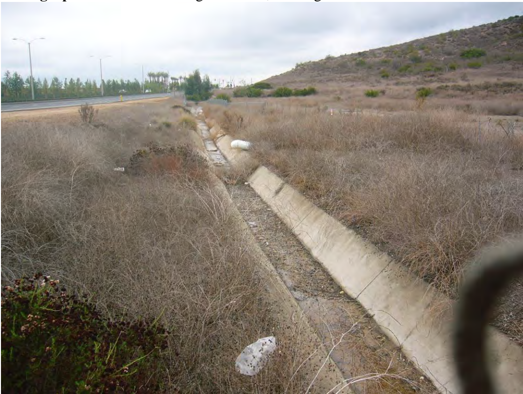
Photograph 2: Portola Drainage Channel, looking west.
