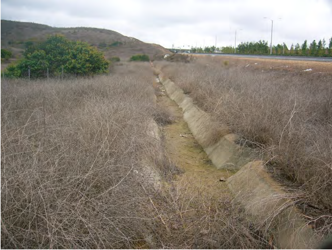
Photograph 1: Portola Drainage Channel, looking east.
