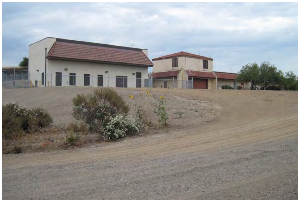
View of non-urban industrial area at the Baker Raw Water Pumping Station.
