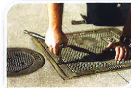
Grease Interceptor is Opened for Inspection
