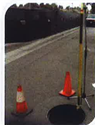
A Probe is Used to Measure the FOG Accumulation in a Grease Interceptor
