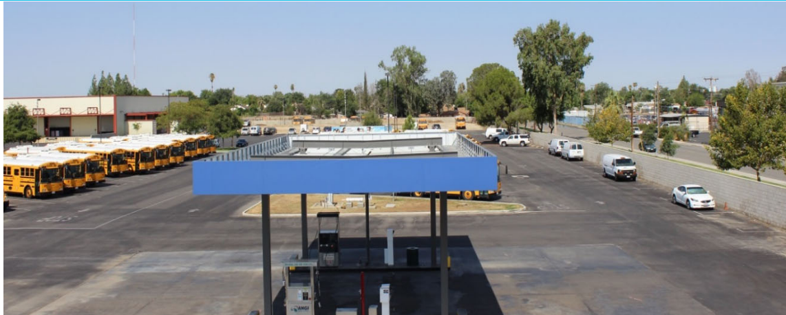
Overview of CNG Fueling Facility
