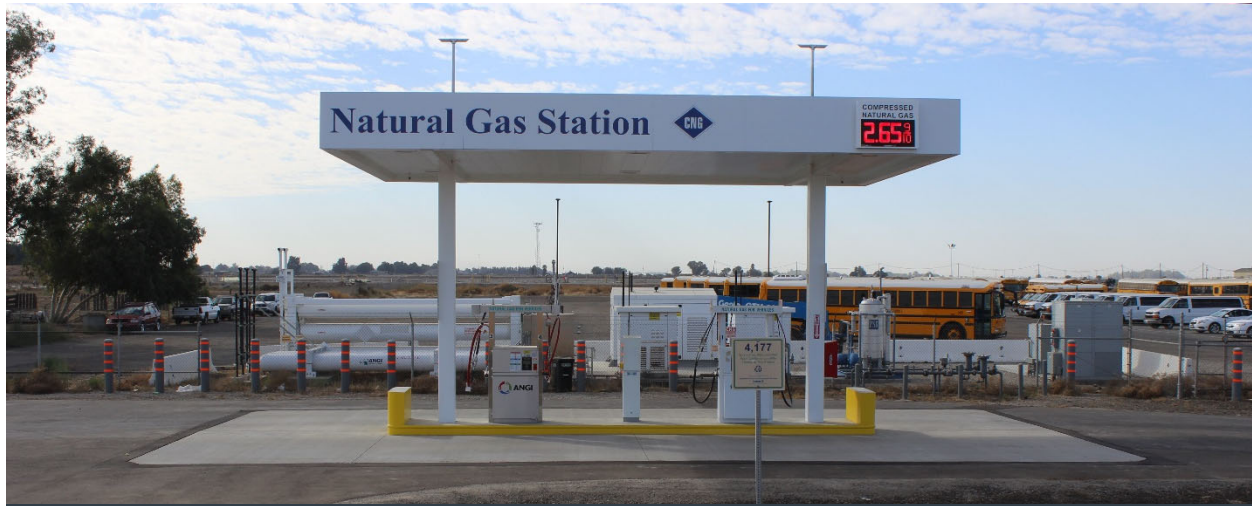
Lemoore Union High School CNG Fueling Station
