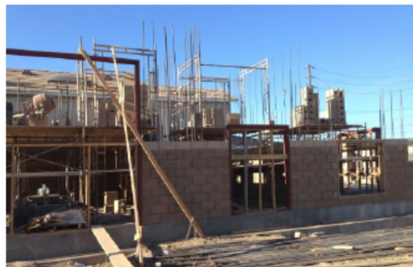
Orange Park Acres Well No. 1 Construction
