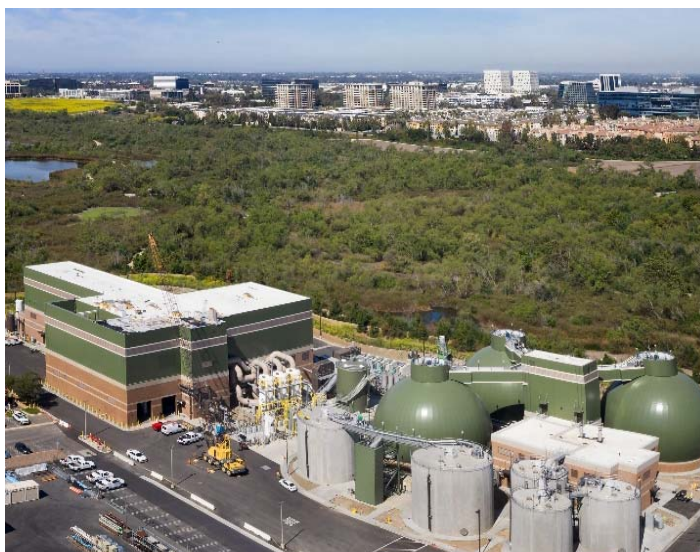
Biosolids and Energy Recovery Facilities
