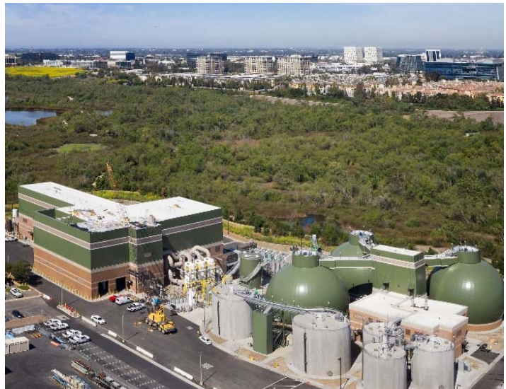
Biosolids and Energy Recovery Facilities
