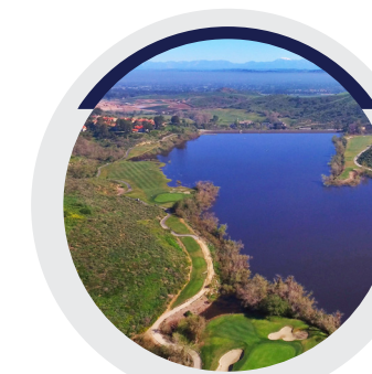
Sand Canyon Reservoir is one of four IRWD seasonal recycled water storage reservoirs.
