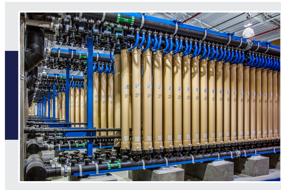
Microfiltration tubes inside the Baker Water Treatment Plant, a 28.1-million-gallon-per-day drinking water treatment facility in Lake Forest. The plant was a joint regional project by five south Orange County water districts and went online in early 2017. The Baker Water Treatment Plant is managed and owned by IRWD.
