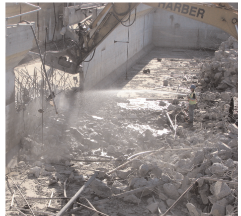
Demolition of the old aerobic digesters at the Michelson Water Recycling Plant was necessary before new construction could begin.
