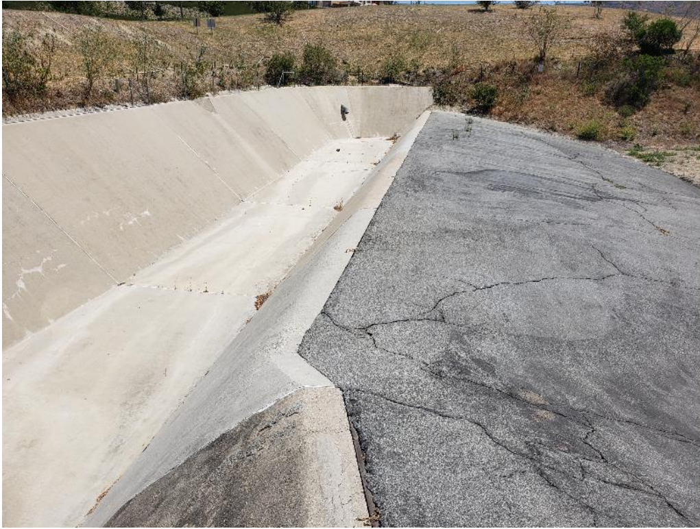
3. Spillway approach, weir, and side channel.
