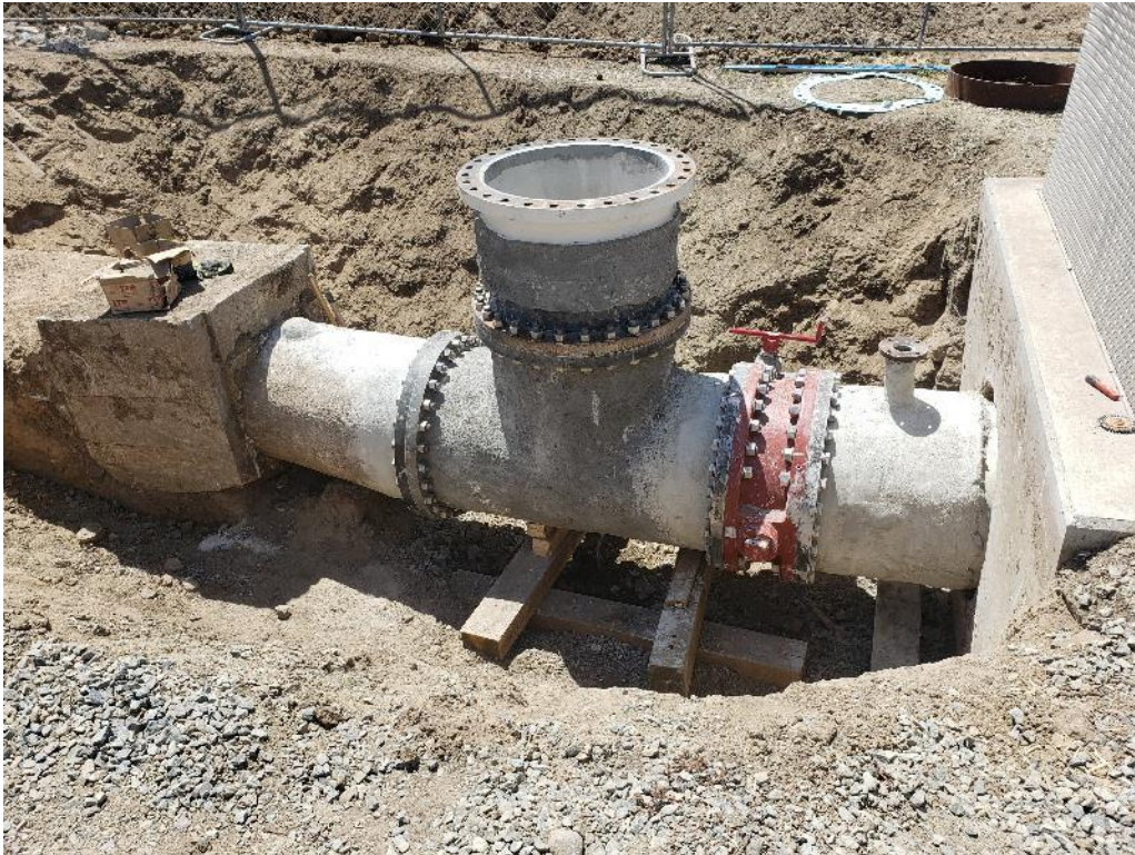
6. New manway and relocation of valve (red).
