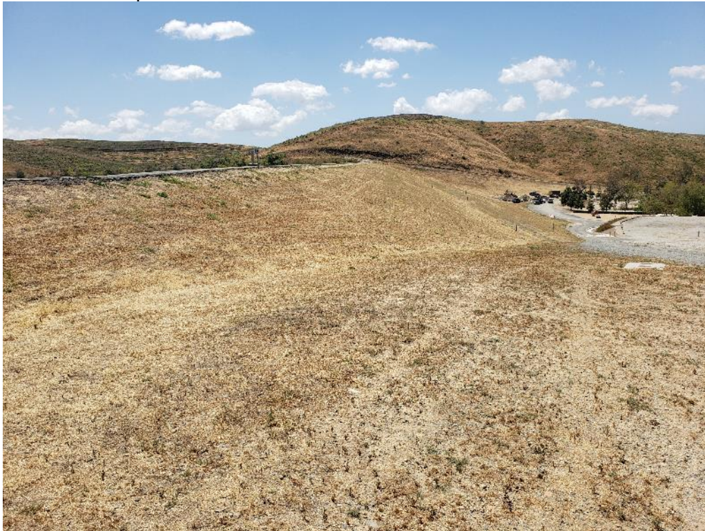
2. Downstream face of the dam observed from the right abutment.
