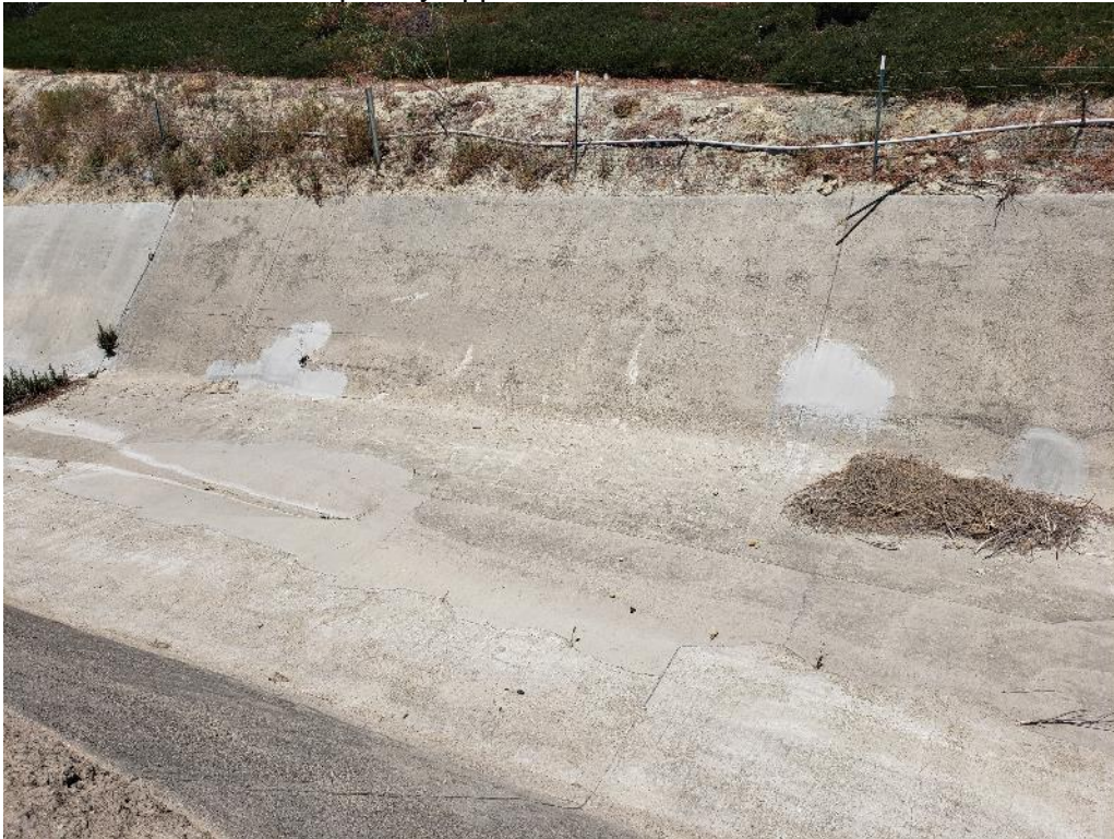
4. Repairs to the spalls with exposed wire mesh reinforcement.
