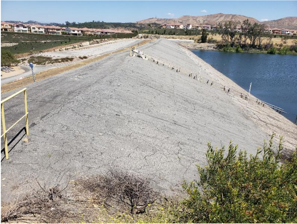
1. Upstream face of the dam observed from the left abutment.
