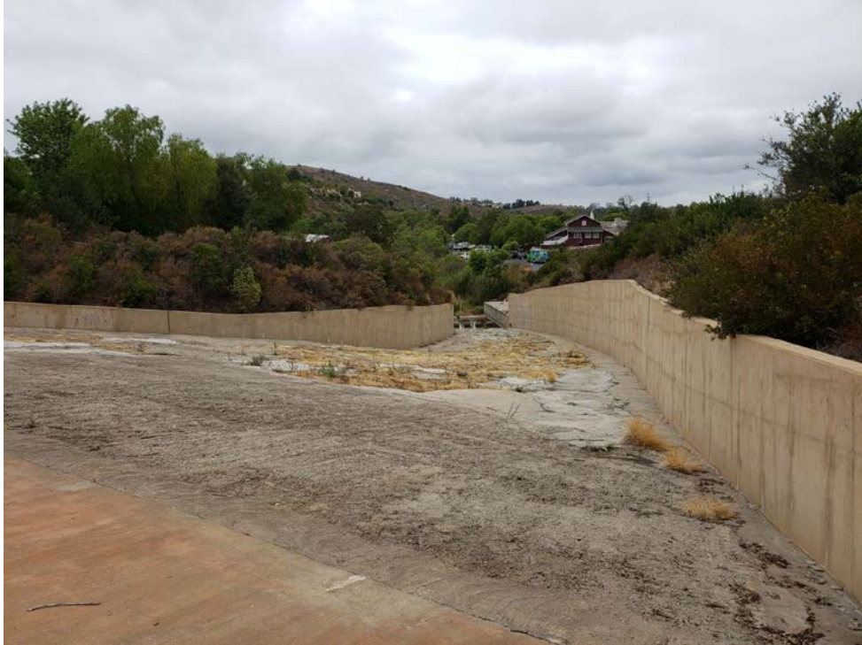
Looking downstream the spillway channel.
