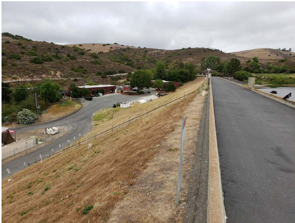
View of the crest and downstream slope.
