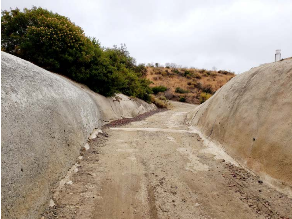
The spillway was open and clear.
