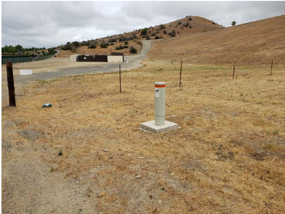
New piezometer installed during the exploration work.
