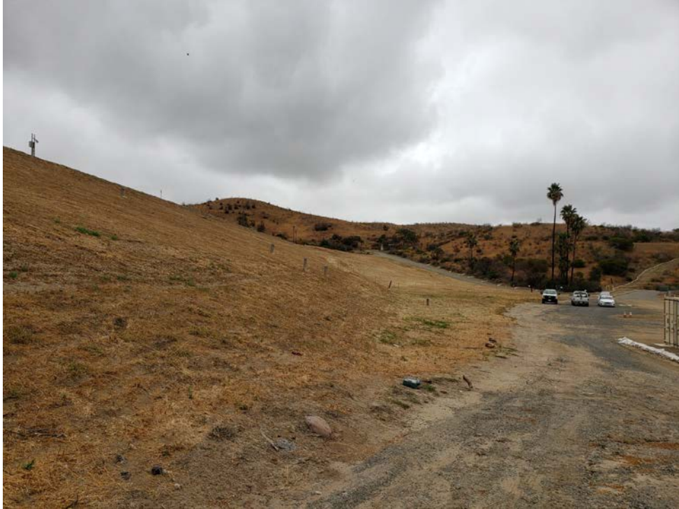
View of the downstream slope and toe area.
