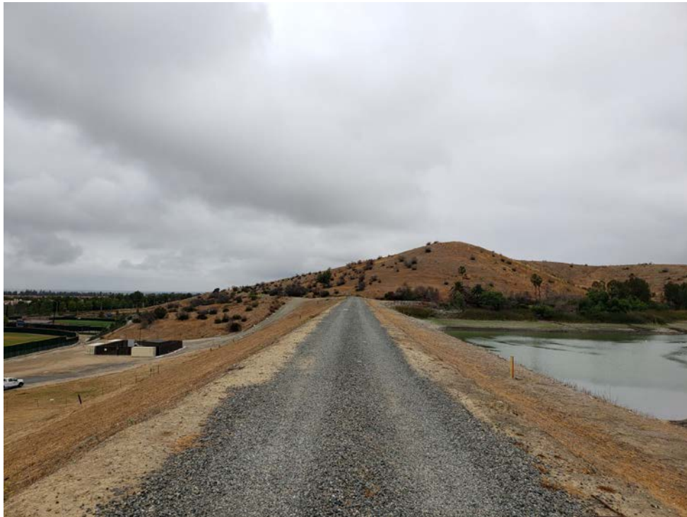
Looking across the crest of the dam.
