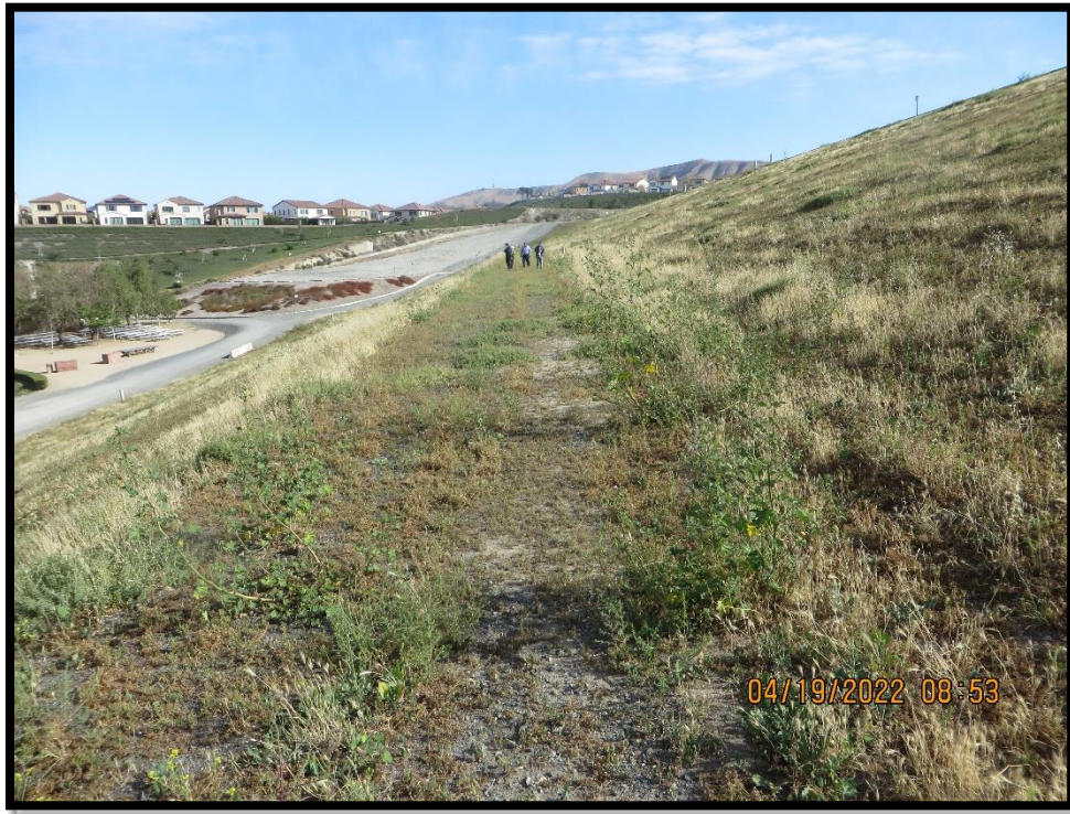
Photo 5) Downstream bench looking towards right abutment.
