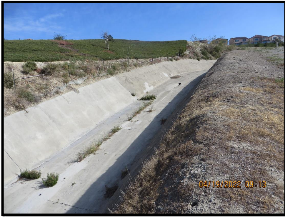
Photo 11) Spillway channel looking upstream. Note white areas that were recently repaired.
