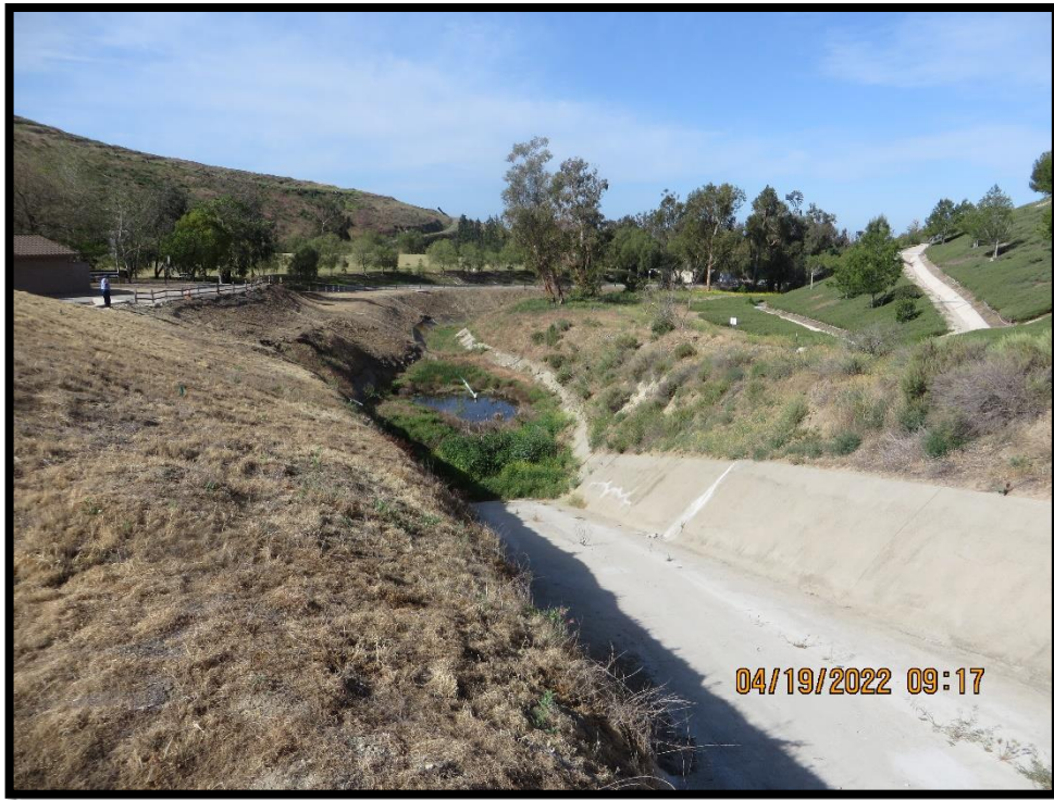
Photo 12) Spillway stilling basin looking downstream. Note minor vegetation.
