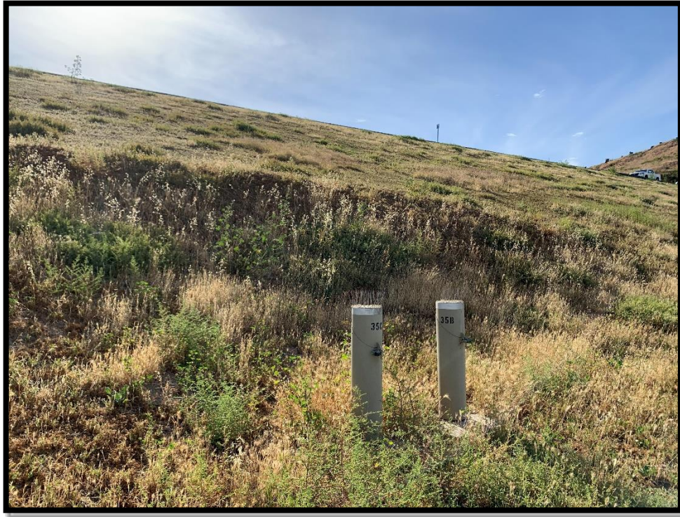
Photo 7) Piezometer location along downstream face at bench looking towards left abutment.
