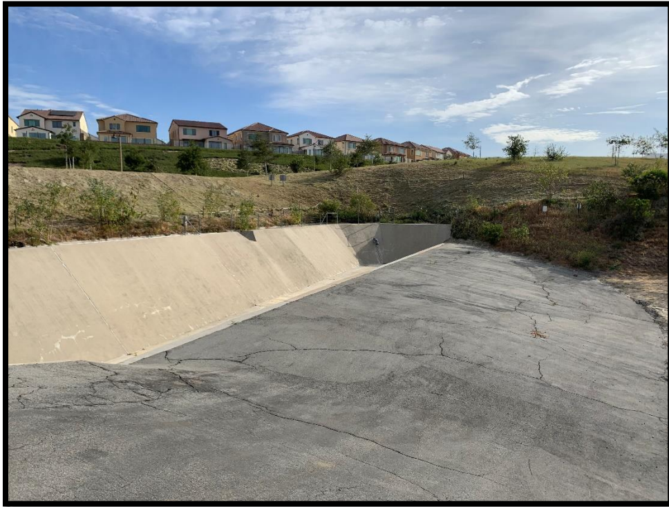
Photo 8) Spillway control section and channel upstream.
