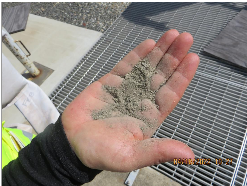
Photo 21) Typical sedimentation sample (after drying) taken from seepage collection drain.
