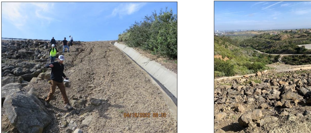
Photo 10) Looking up and down left groin area, respectively.
