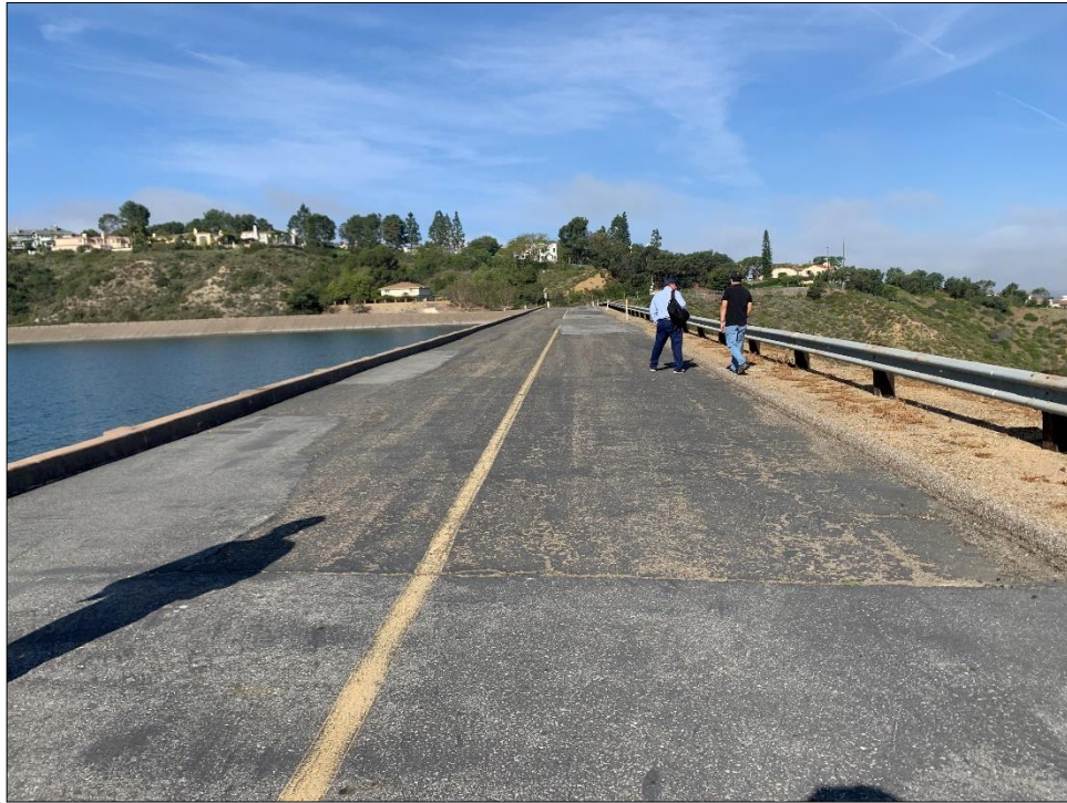
Photo 5) AC paved crest looking towards the left abutment.
