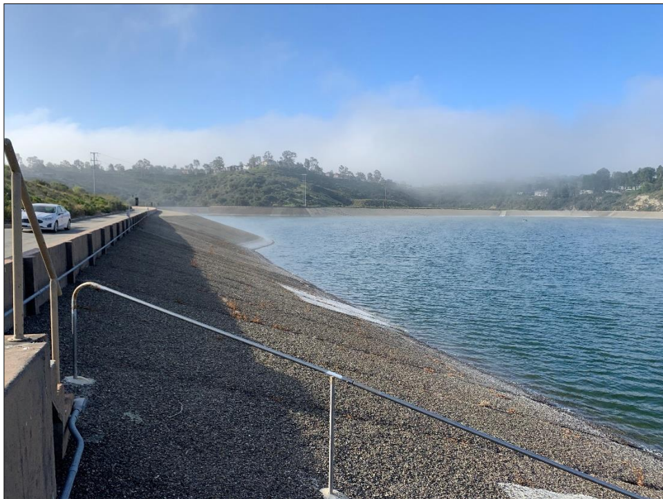
Photo 2) View of eastern slope of AC-lined reservoir.
