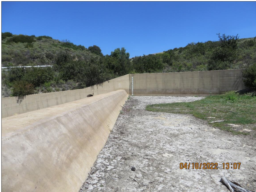
Photo 8) Close view of the spillway control ogee section and approach.
