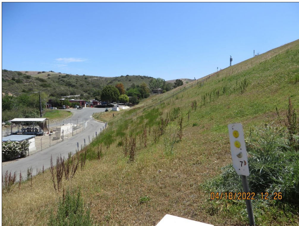
Photo 6) Downstream face looking towards the right abutment.
