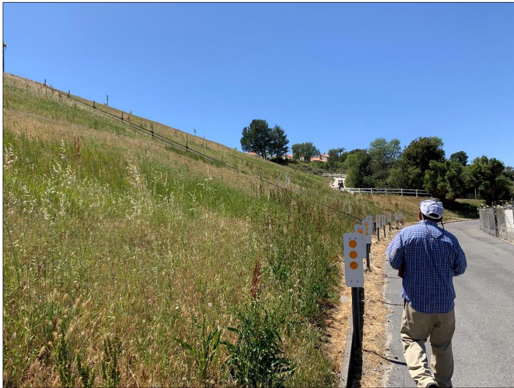
Photo 5) Downstream face looking towards the left abutment.
