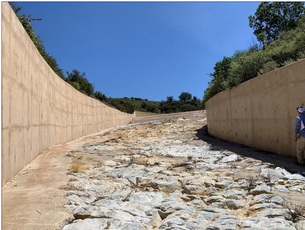
Photo 10) Spillway channel concrete walls and rock floor looking upstream.
