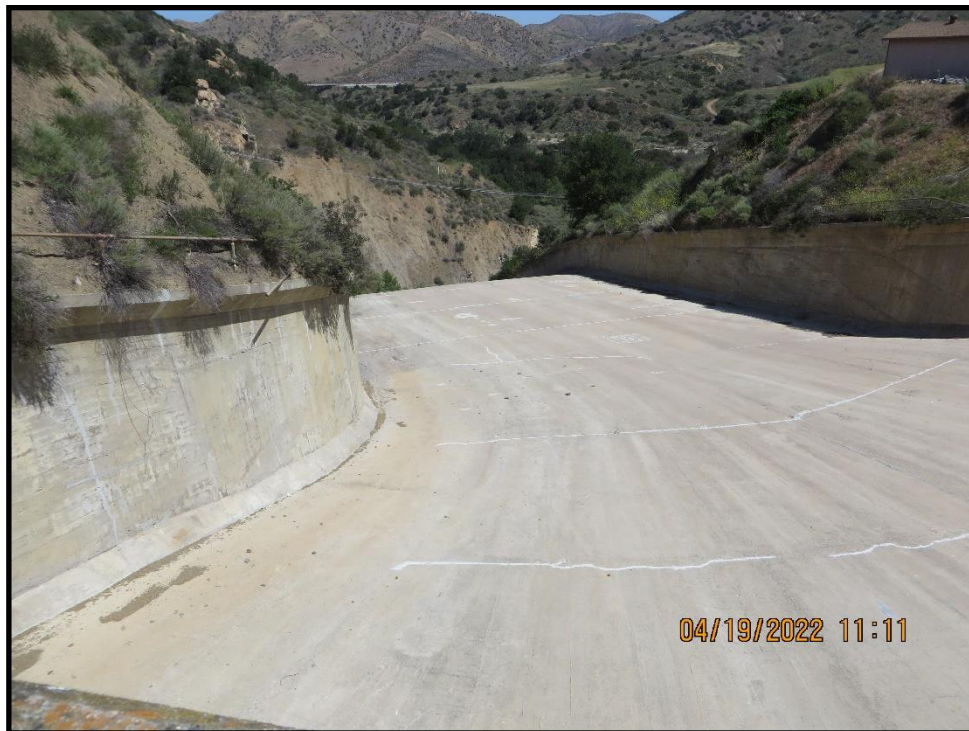
Photo 8) Spillway chute, looking downstream.
