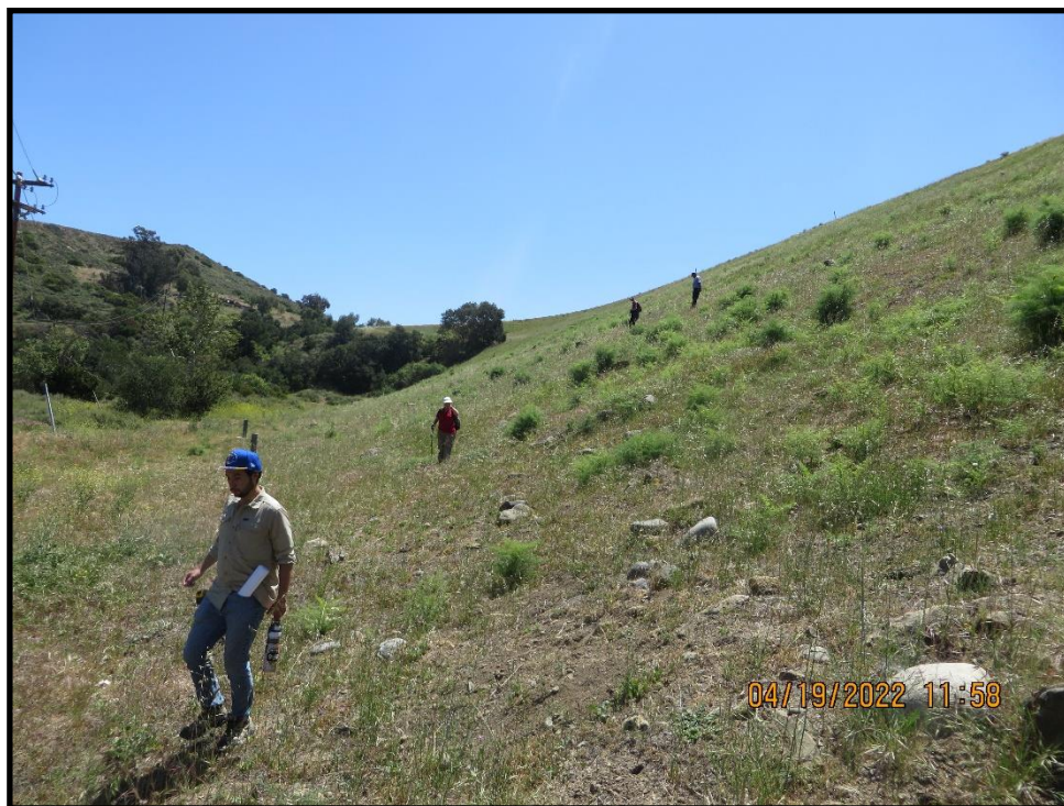
Photo 16) Downstream slope looking up to crest and toward right end of dam. Note regrowth of brush vegetation.
