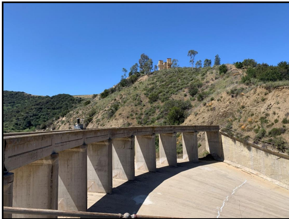
Photo 6) Spillway concrete bridge, piers, and chute looking toward left abutment.
