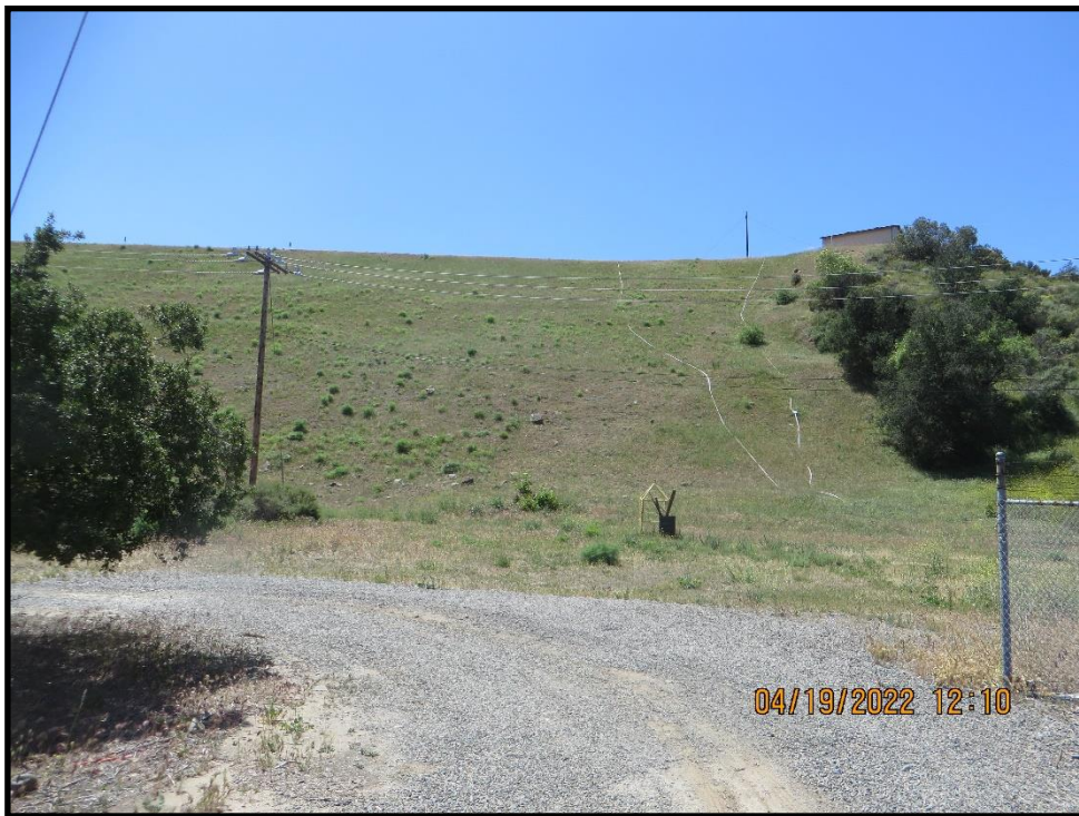
Photo 18) Old water irrigation lines coming down downstream slope near left abutment. Note regrowth of brush.
