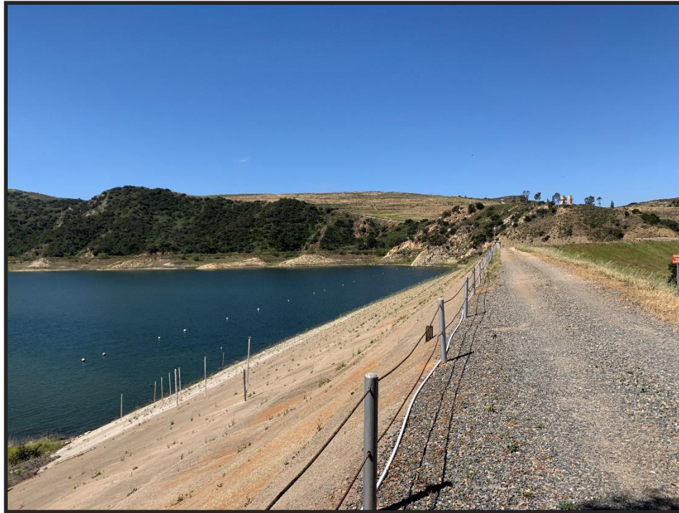
Photo 1) Crest and upstream face.
