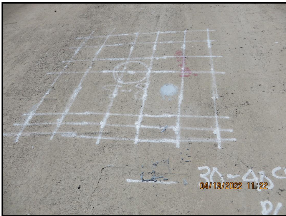
Photo 12) Location of previously drilled boring hole at spillway.
