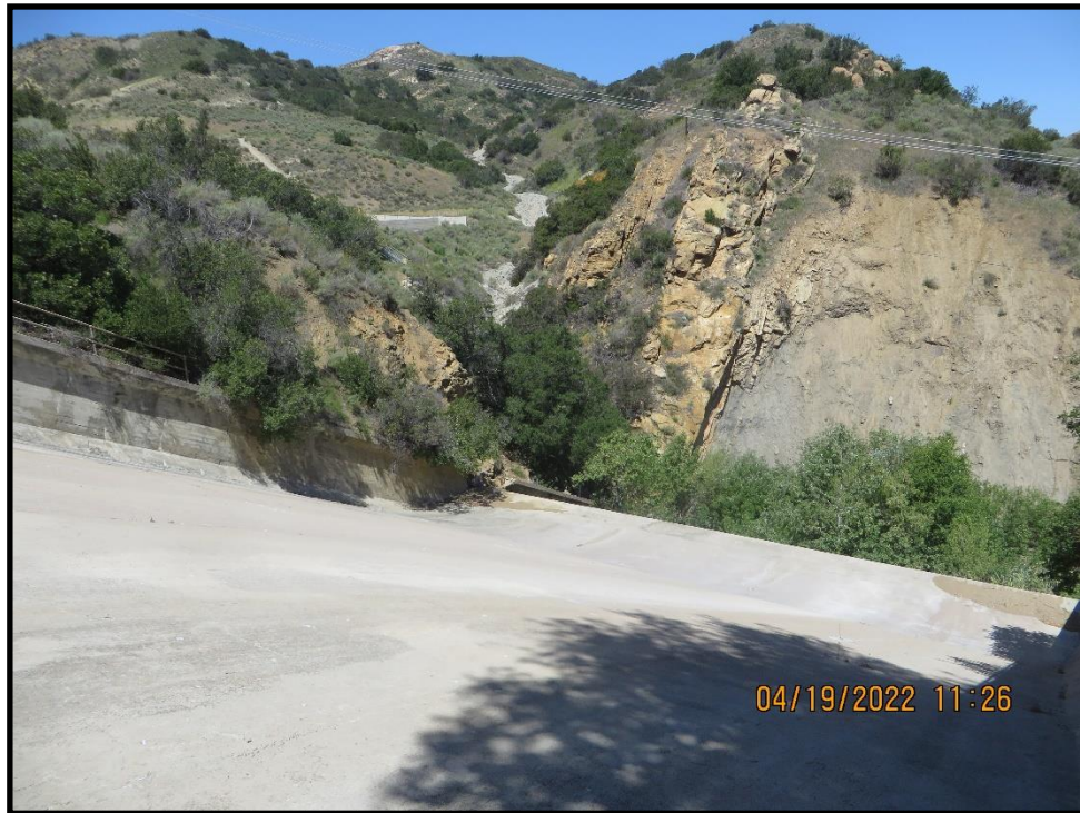
Photo 13) Spillway chute looking downstream.
