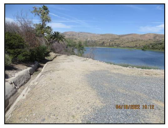
Photo 4) Old ditch and vegetation growing on right upstream groin riprap area.
