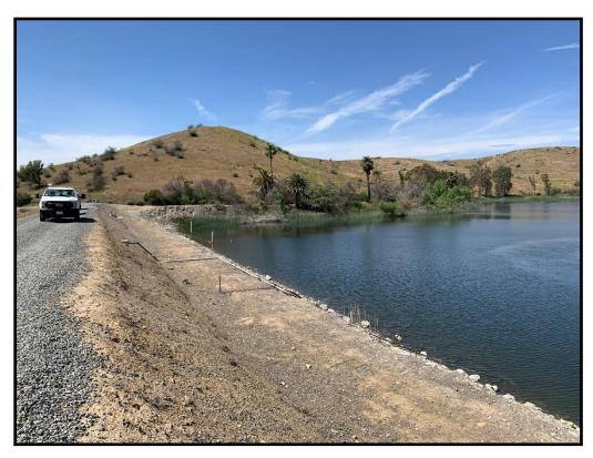
Photo 1) Crest and upstream face looking towards right abutment showing bench.
