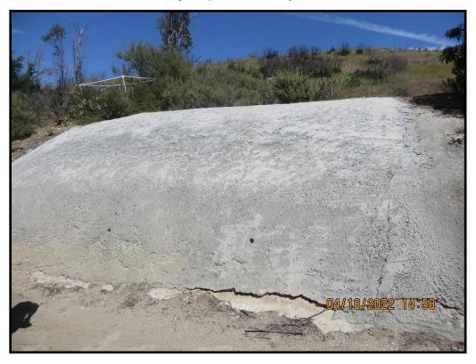
Photo 8) Deterioration at spillway channel looking east.
