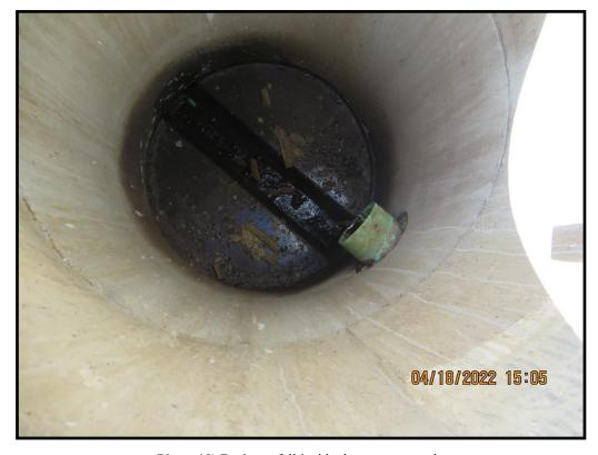
Photo 10) Drain outfall inside the seepage vault.
