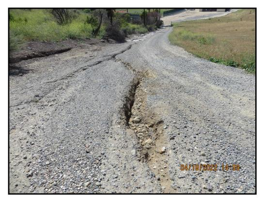
Photo 11) Erosion rills at left abutment access road.
