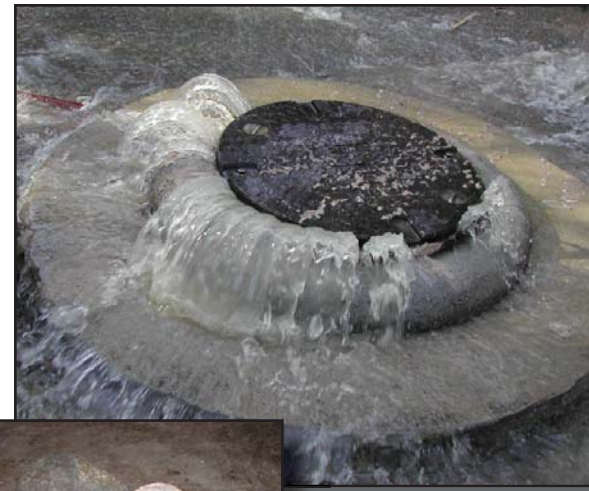
Rocks, such as these, at left, can cause a sewer spill, like the one pictured above.
